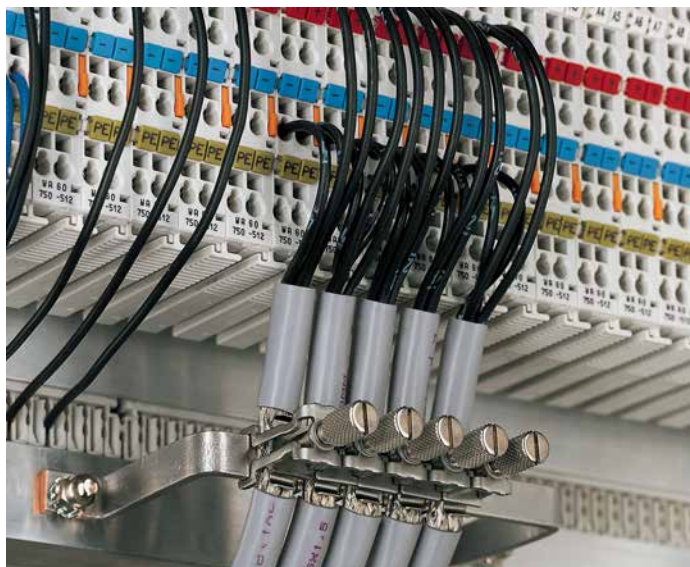
Figure 20: Application of the WAGO Shield Connecting System
